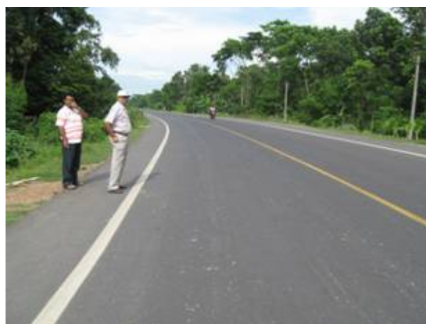
road view after 6 months
