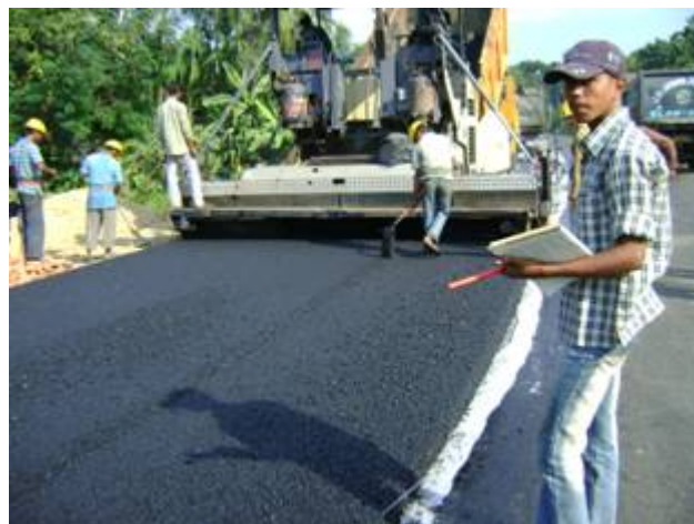
Paving with asphalt concrete
