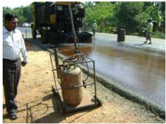
Spraying Tack Coat
