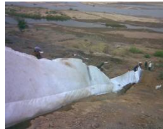
Installation of Viadrain in slope trench
