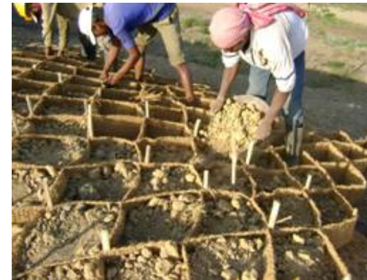
Installation of Coir Geocells and soil
