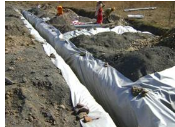
Fibertex F-25 NW Geotextile for Trench drains
