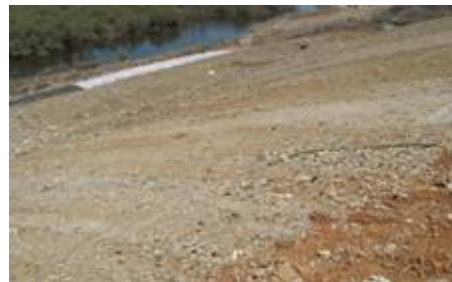
Soil Regularization layer
