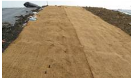
Top Soil and Coir Erosion control Blanket
