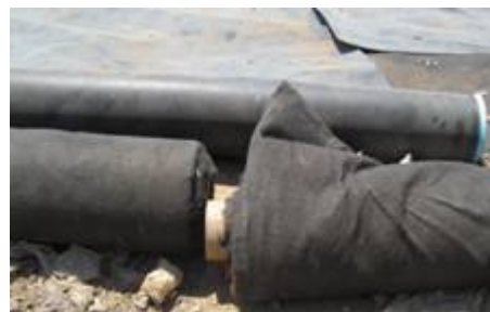
Geomembrane and Geotextile
