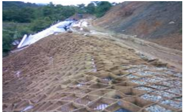
Installation of all items
