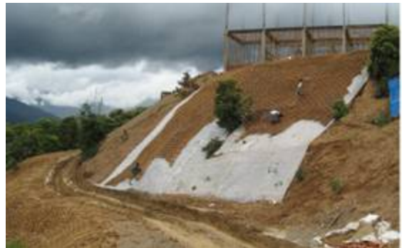
Installation of Grids and Coir Geocell
